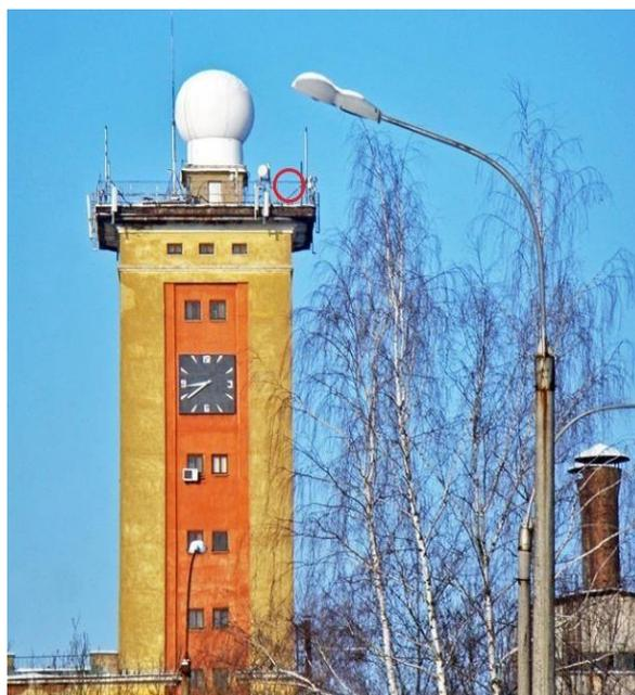
Figure 2. Placement of preparations (samples) at a distance of 46 m from the ground. Place of the attachment indicated by a circle.
